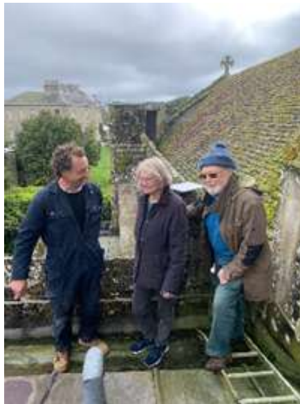
Inspecting damage to the roof of the North Transept May 2024
